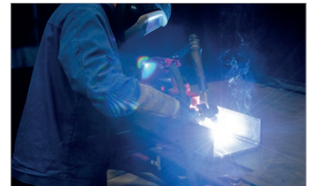
Welding in narrow spaces (min. width 200 mm)
