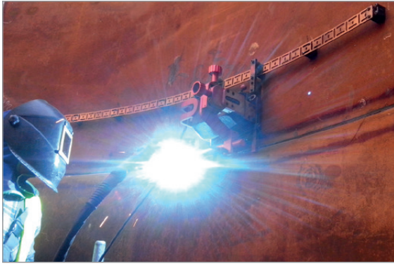
Flexibele rails lengte 1.88 meter (6.1ft) Minimale radius is 1,0 mtr (3,3 ft) PRW-0466-50-01-01-0
