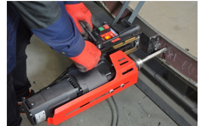
Out of position drilling
